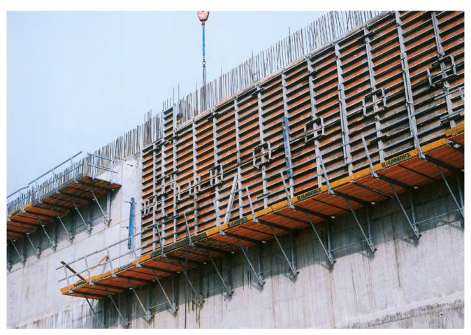
▶ Withstands up to 2.00 kN/m² in combination with a 5.40 m high formwork and up to 6.00 kN/m² without formwork
