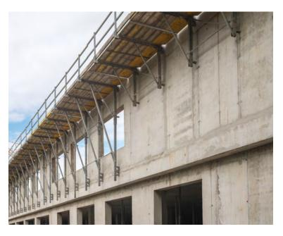
By using the KG bearer bars and KG suspension bars, large wall openings are easily overcome
