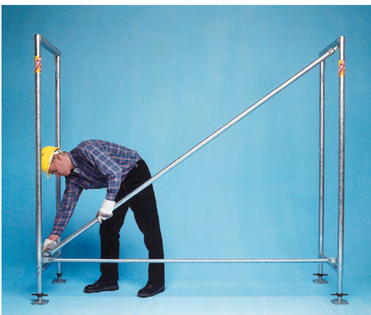
► Safe and inevitably plumb-vertical erection already after assembly of the first bay
