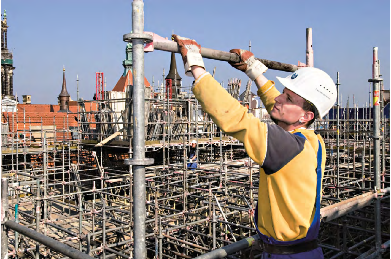
▶ Safe one-man assembly at any height due to the upturned edge on the connection cups
