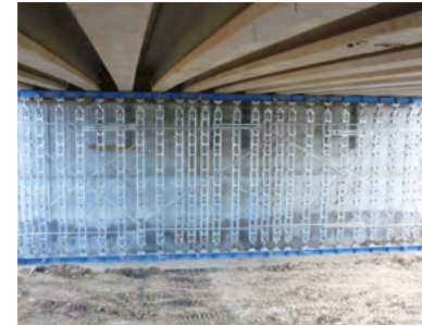
Heavy duty shoring
