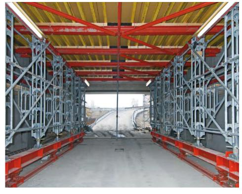
Load-bearing frame props used as shoring solution for an unobstructed site underpass
