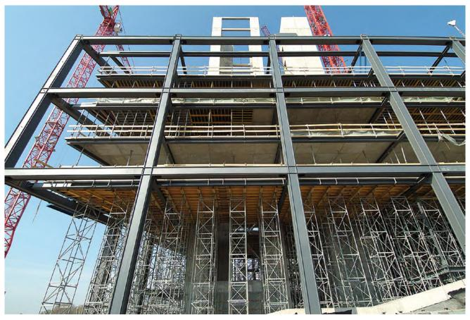
▶ High load capacity of 180 kN per tower even with small base dimensions (1.00 m x 1.00 m)
