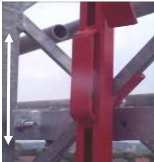
Fig. 34: Installation of the floor limit switch plate
