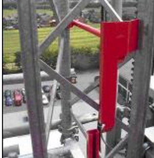
Fig. 32: Installation of the upper limit switch plate
