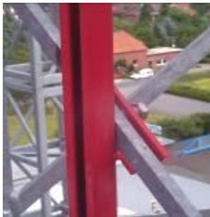
Fig. 33: Installation of the floor limit switch rail
