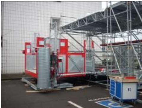
Fig. 17: Pre-assembled platform group in front of building wall
