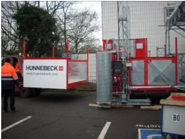
Fig. 18: Position the standard loading platform
