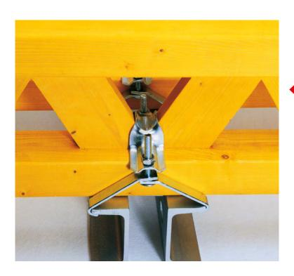
Standard walers from 1.0 – 3.0 m for element widths in 25 cm increments make object-related element dimensions simple for planning and forming operations
