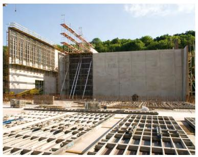
▶ By using facade soldiers, the 16.73 m high walls of a terminal were shuttered in two pouring cycles instead of three.
