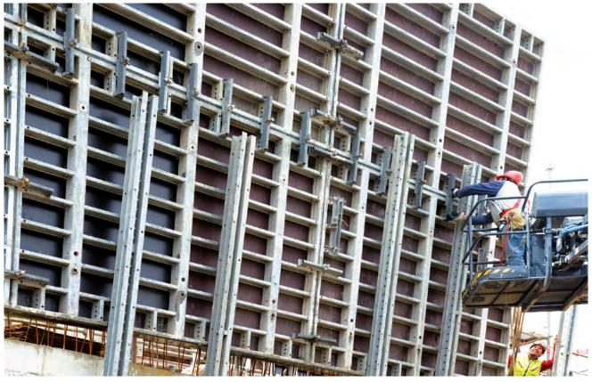
A special solution: Facade walers are used to ensured back anchoring of the horizontal loads and to enable the exact alignment of the MANTO formwork in a desired inclined position.
