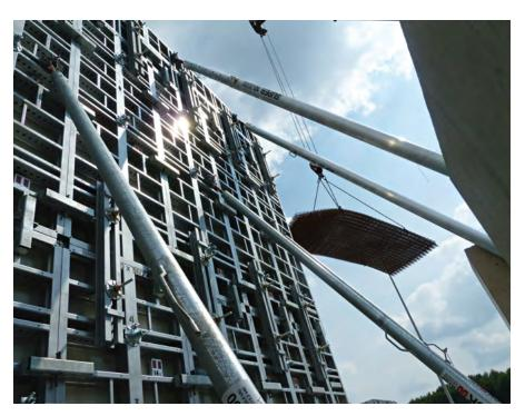
▶100 kN/m² concrete pressure throughout the system for new SCC and liquid concrete types
