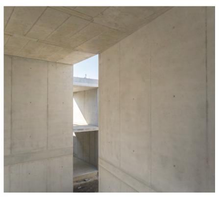
Neatly aligned tying and joint grid possible, no matter if the panels are used in upright or horizontal positions
