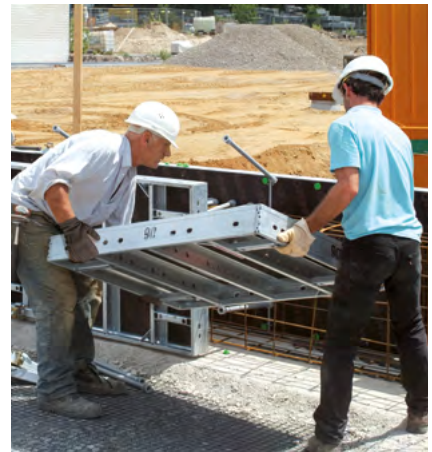
▶ RASTO as foundation formwork
