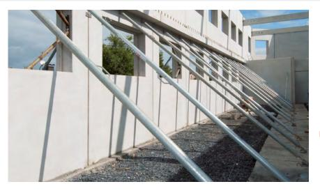
Great load-capacity to self-weight ratio comprising five strut types with extension lengths from 2.05 m – 10.25 m
