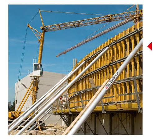
The Super 10 is an aluminium strut, which is ideal for larger tasks. An additional advantage: since the threaded part of the Hünnebeck aligning struts are protected with a cover, they always stay clean and can be easily used and remain ready for use, even after multiple applications.
