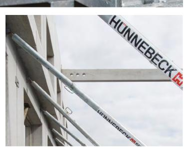
Simplified and convenient dismantling due to the separation of strut from the quick-action fastener
