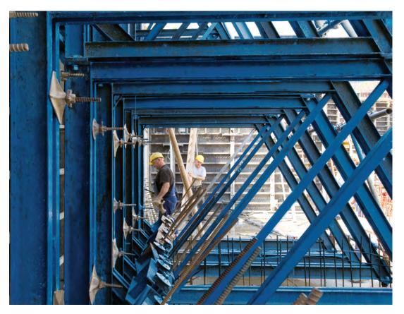
▶ High strength: support frames can withstand a maximum concrete pressure of up to 60 kN/m<sup>2</sup>
