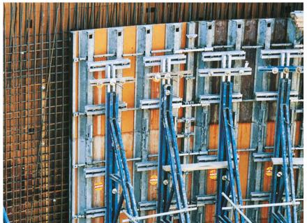
Distances between support frames can be adapted according to plan
