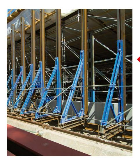
Support frames can also be used in a special application to stabilise MODEX scaffolding against horizontal forces
