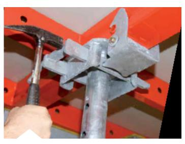
Specially developed folding heads with self-securing pins make it effortless to
