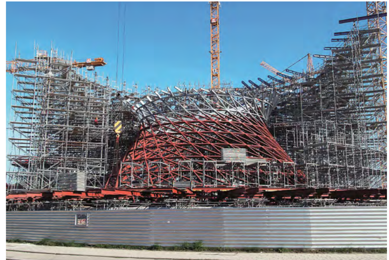
▶ BOSTA 70 is compatible with MODEX. Here it is used in combination to form a star-shaped corset that was used to deflect loads.
