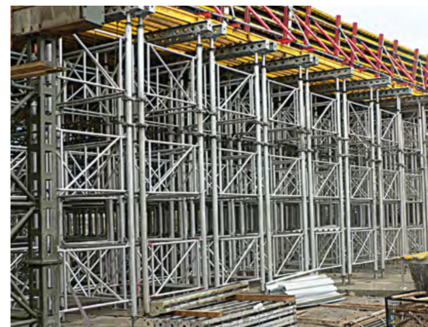
▶ Bridge deck and parapet shoring
