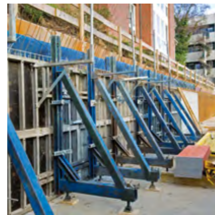
▶ Distances between support frames can be adapted according to plan
