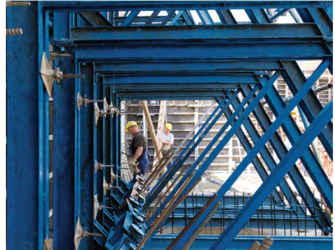
▶ High strength: support frames can withstand a maximum concrete pressure of up to 60 kN/m 2
