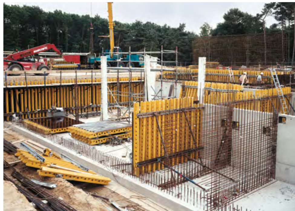
▶ Free choice of plywood provides flexibility in terms of the required quality of concrete surface
