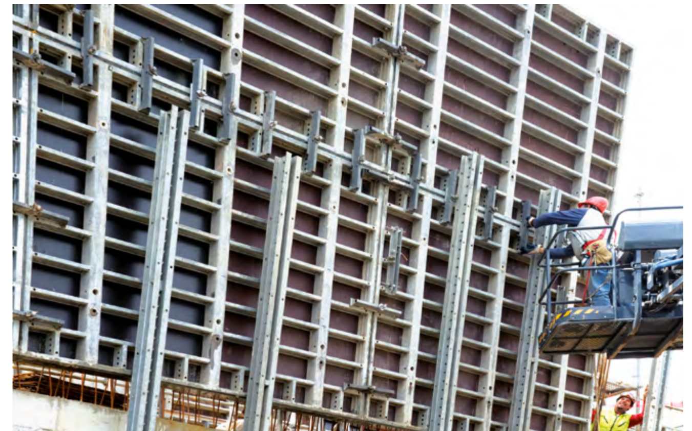
▶ A special solution: Facade walers are used to ensure back anchoring of the horizontal loads and to enable the exact alignment of the MANTO formwork in a desired inclined position.
