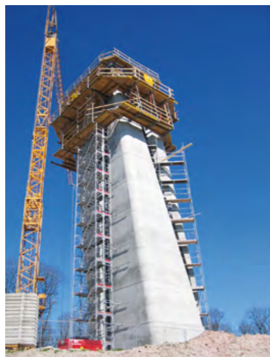
Formwork can be rolled back from concrete by means of move-off unit
