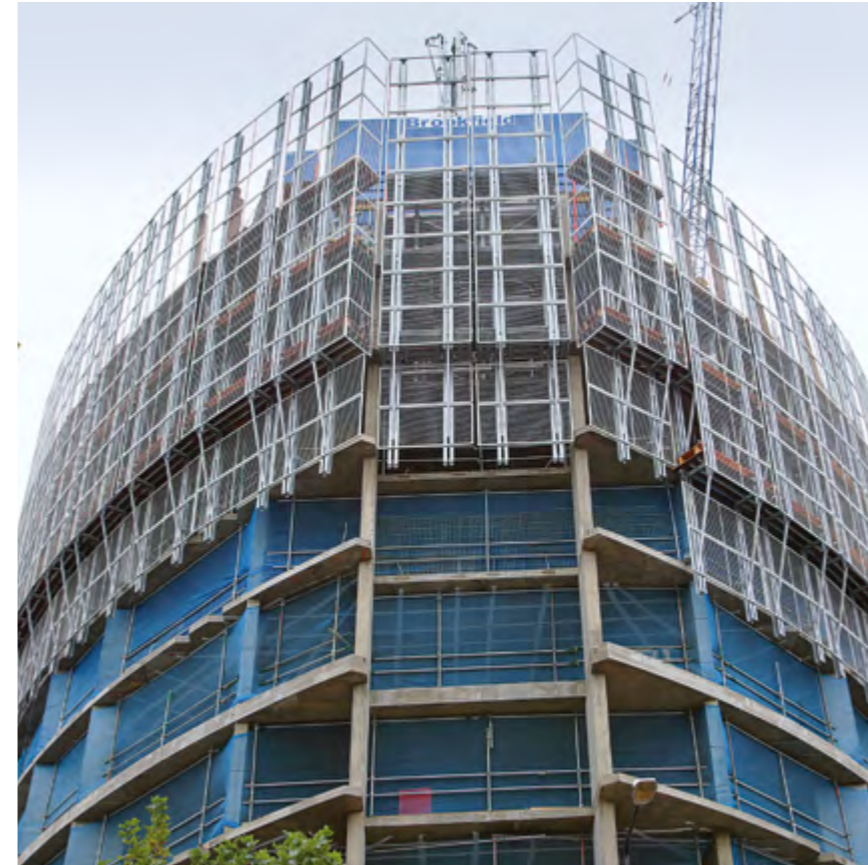
▶ Complex architecture easily accommodated
