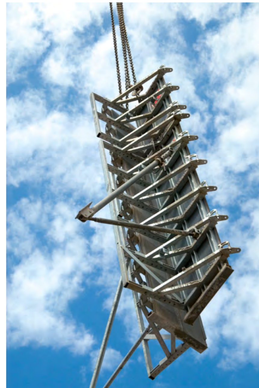
▶ Moving complete units with a single crane pick. All accessories are firmly secured to the element
