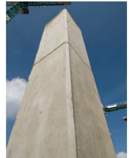
▶ Superb concrete finish and more re-uses thanks to the plastic-coated plywood
