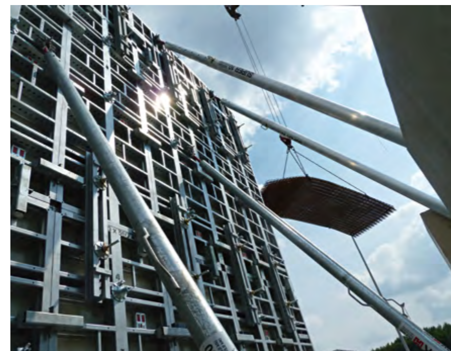
▶ 100 kN/m 2 concrete pressure throughout the system for new SCC and liquid concrete types
