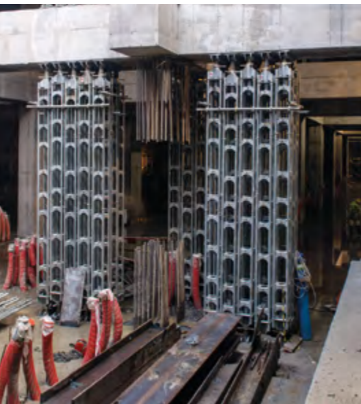
▶ Very high load capacity up to 210 kN even with small base dimensions of only 25 x 25 cm
