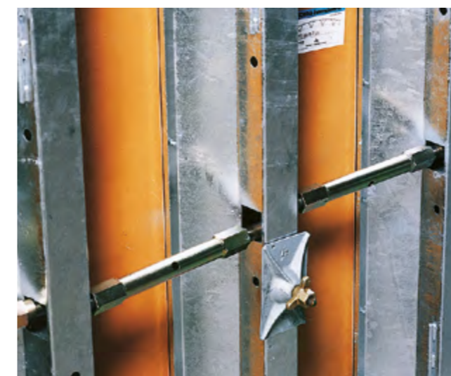
▶ Millimetre-precise radius adjustment using turnbuckles and fine-tune alignment thanks to lever edge on profiles
