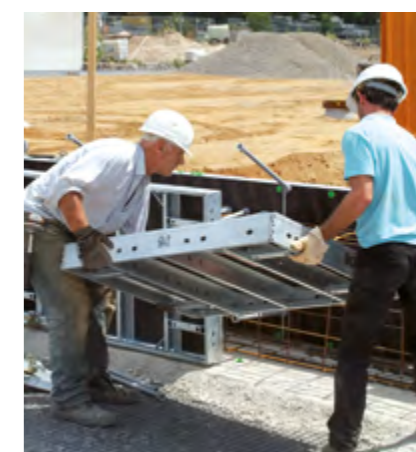
▶ RASTO as foundation formwork
