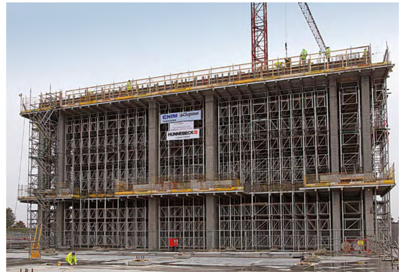
▶ Heavy-duty capacity of up to 140 kN reduces the amount of equipment required
