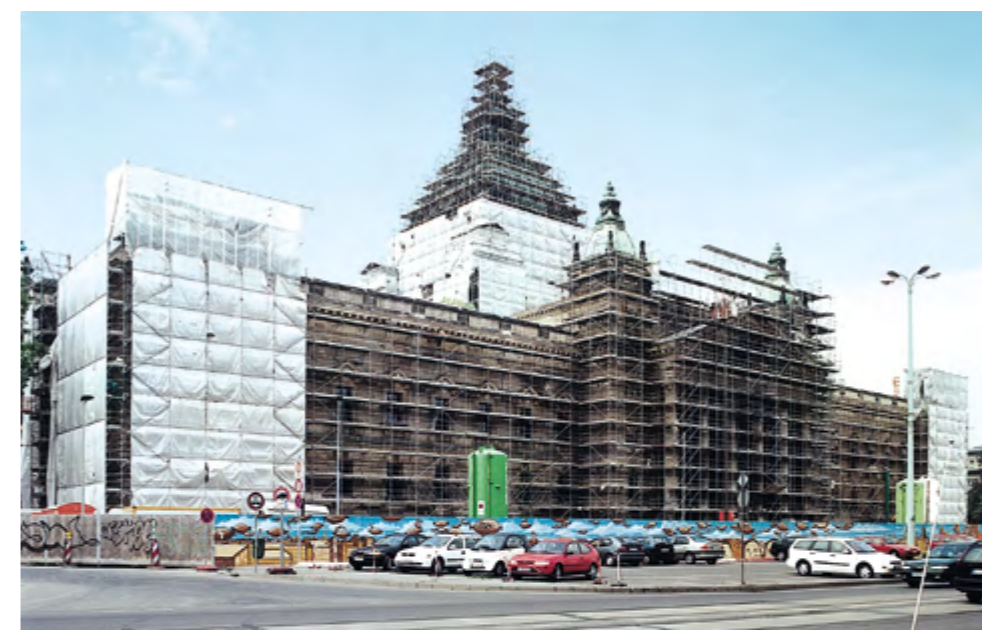
▶ BOSTA 100 is the ideal scaffold whenever additional space is required to move around and temporarily store materials
