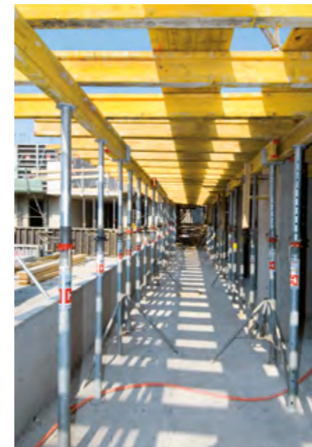
▶ Optimal prop arrangement for the given loads as a result of variable distances between props
