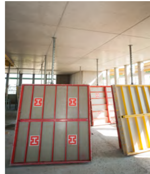
▶ This giant panel measuring 180 x 180 cm has a forming area of 3.24 m 2 .
