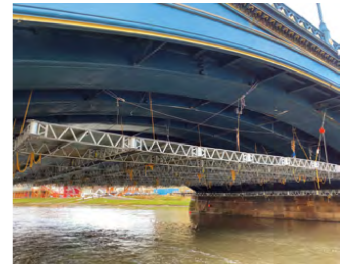
► Trent River Bridge (UK): QuikDeck provides large safety margins thanks to high load capacity of the suspension chains
