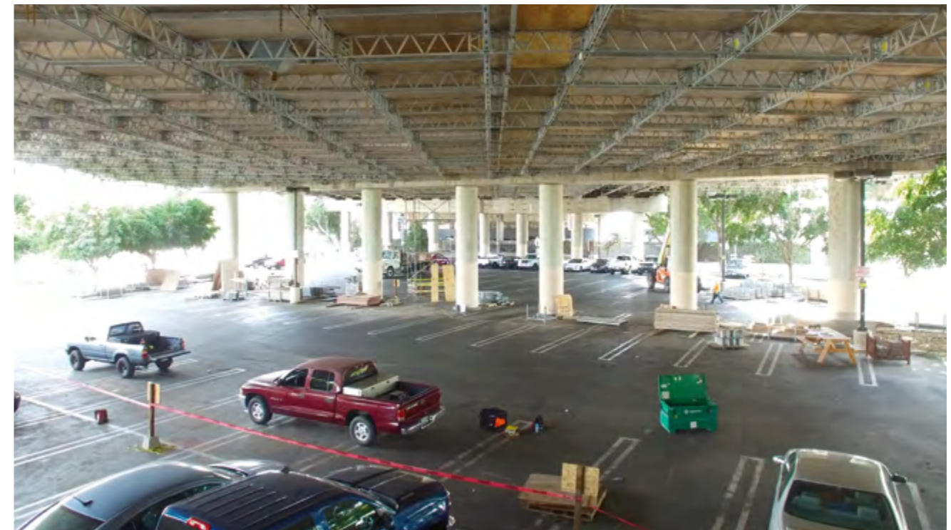
► The QuikDeck suspended platform enables work without interruption, e.g. during bridge renovations. There is usually no need for traffic closures – on or under bridges
