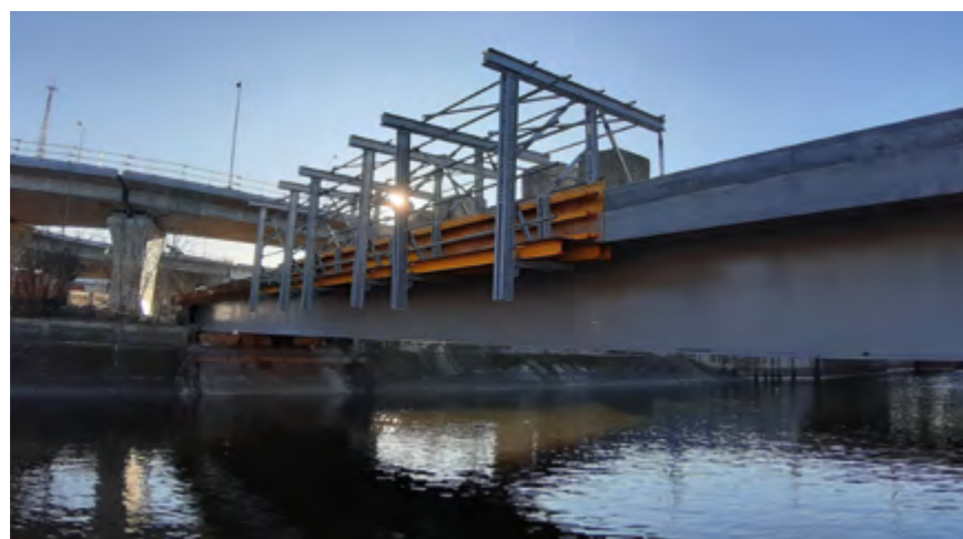
▶ Anchoring to the structure not required
