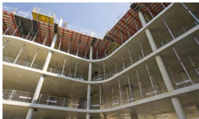
▶ High safety measures due to compatibility with PROTECTO edge guard system
