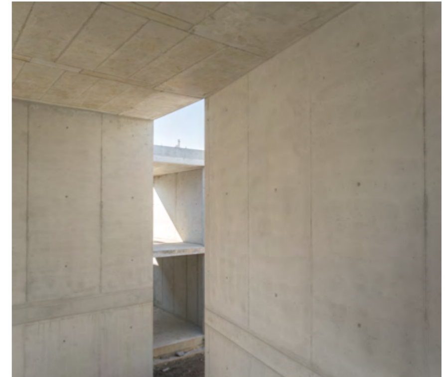
▶ Neatly aligned tying and joint grid possible, no matter if the panels are used in upright or horizontal positions
