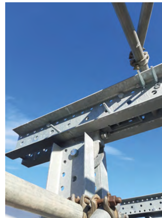
▶ Continuously perforated U-beams for installing the fasteners at any point. This allows the formwork to be used at any desired angle
