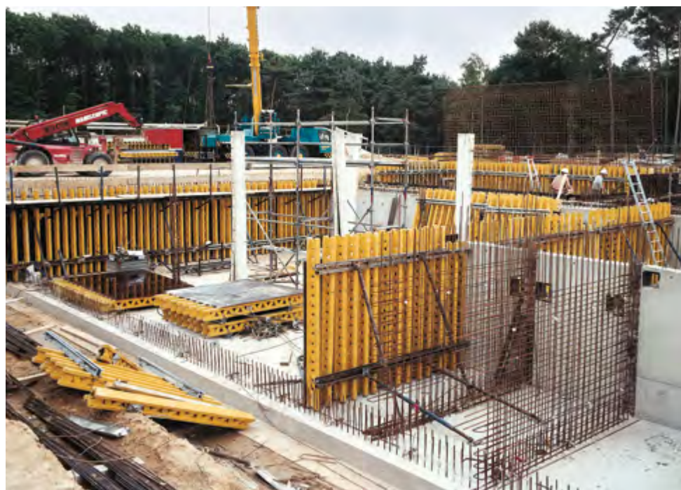
► Free choice of plywood provides flexibility in terms of the required quality of concrete surface
