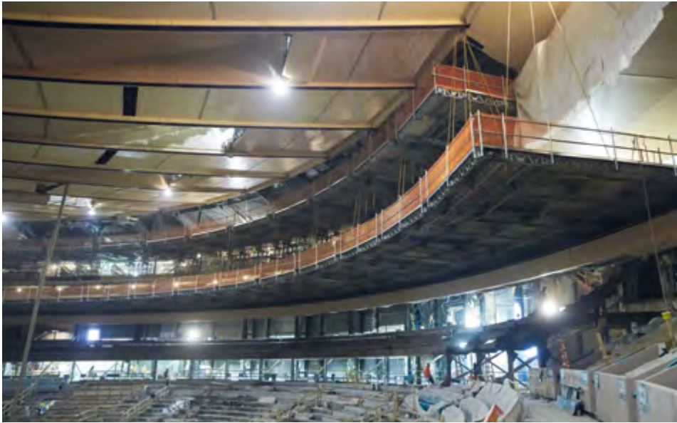
► Madison Square Garden (New York City) During renovation work in Madison Square Garden, Penn Station, which is located underneath and serves as a major transportation hub in New York, had to remain open. QuikDeck was the perfect solution for worker access
