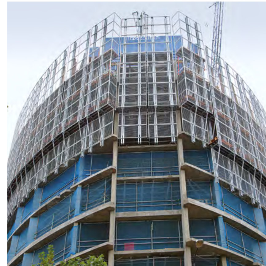
► Complex architecture easily accommodated
