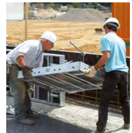
► RASTO as foundation formwork
