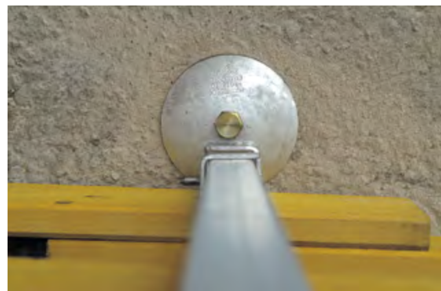
► Screw base joint can easily be fixed to the base slab
