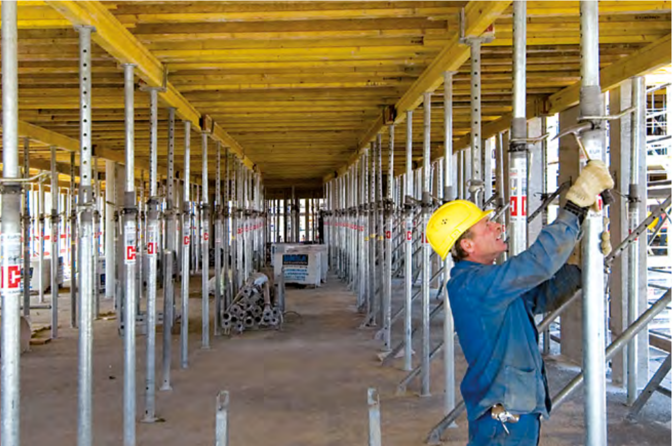
► Stripping is made easier by lowering the forming plane by about 6 cm using the adjustment nut of the steel props
