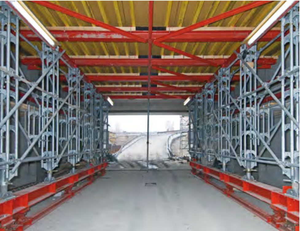
► Load-bearing frame props used as shoring solution for an unobstructed site underpass
