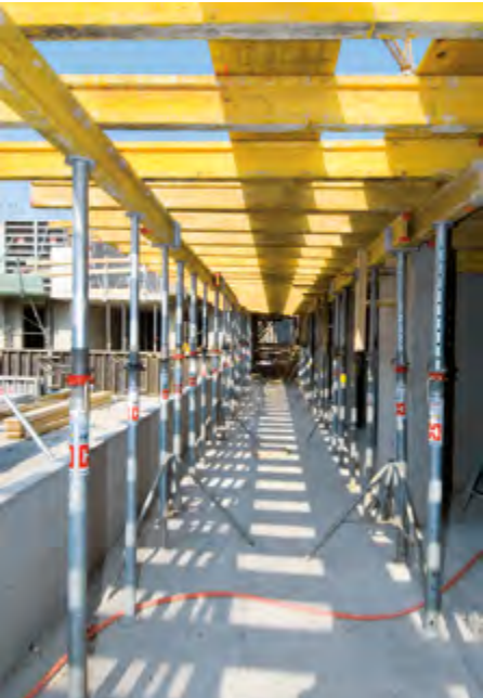
► Optimal prop arrangement for the given loads as a result of variable distances between props
