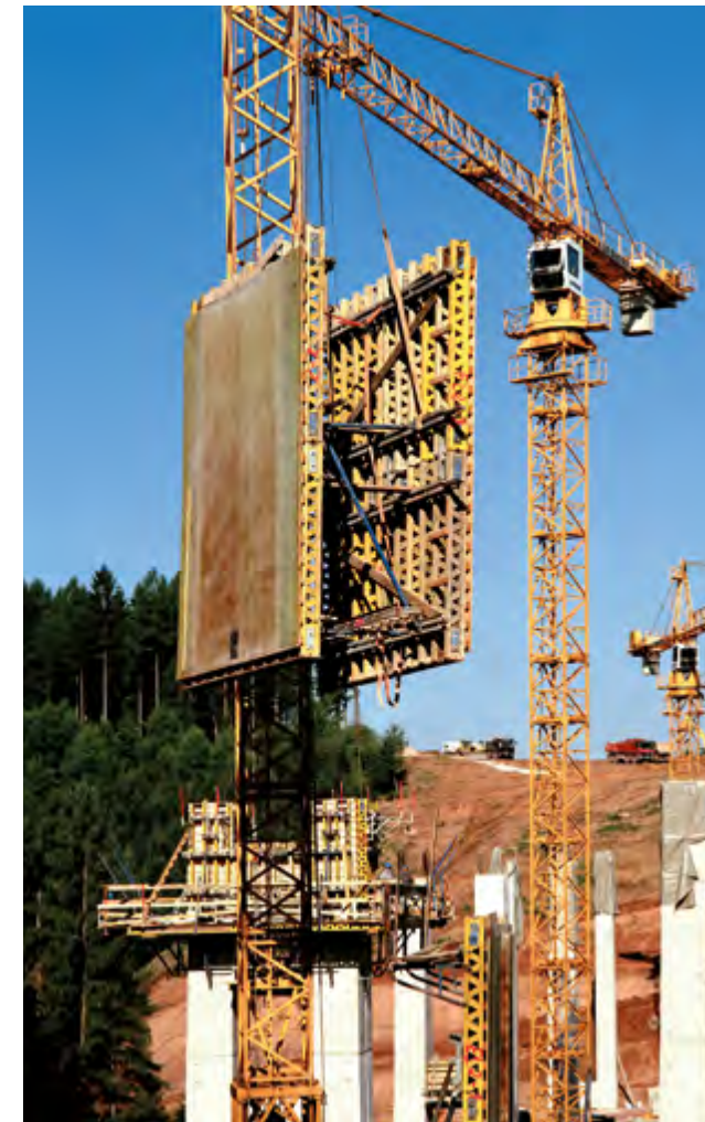
► Easy assembly and disassembly of formwork units enable trouble-free retrofitting in case of frequent changes to the ground plan
