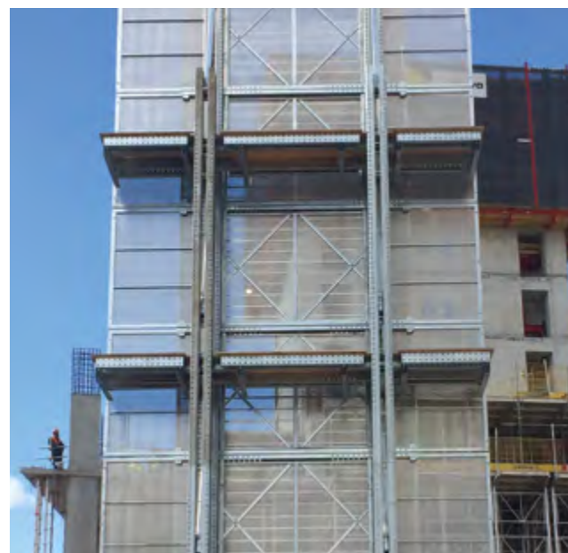
► Multiple floor protection with optional vertical extension
