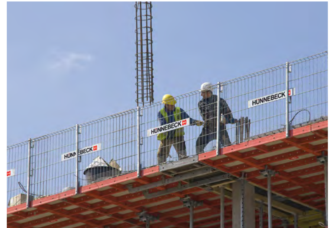
► PROTECTO is compatible with all Hunnebeck slab formwork systems, such as TOPMAX as shown here
