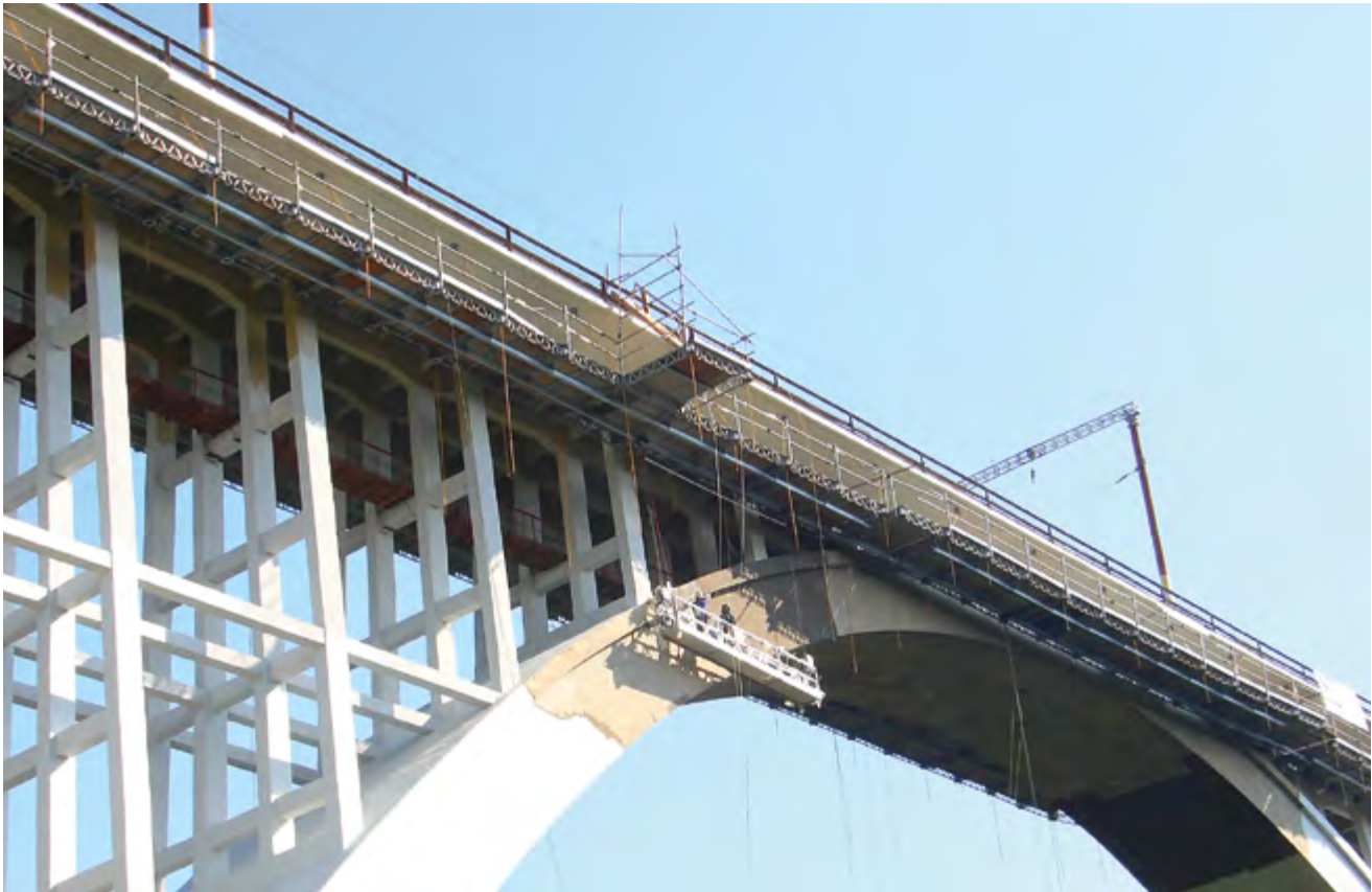
► The QuikDeck platforms suspended from the Romanian railway bridge of Caracău Viaduct provide a consistent, safe working level and replace classic spatial scaffolding. This lowers the costs of bridge maintenance and speeds up the work
