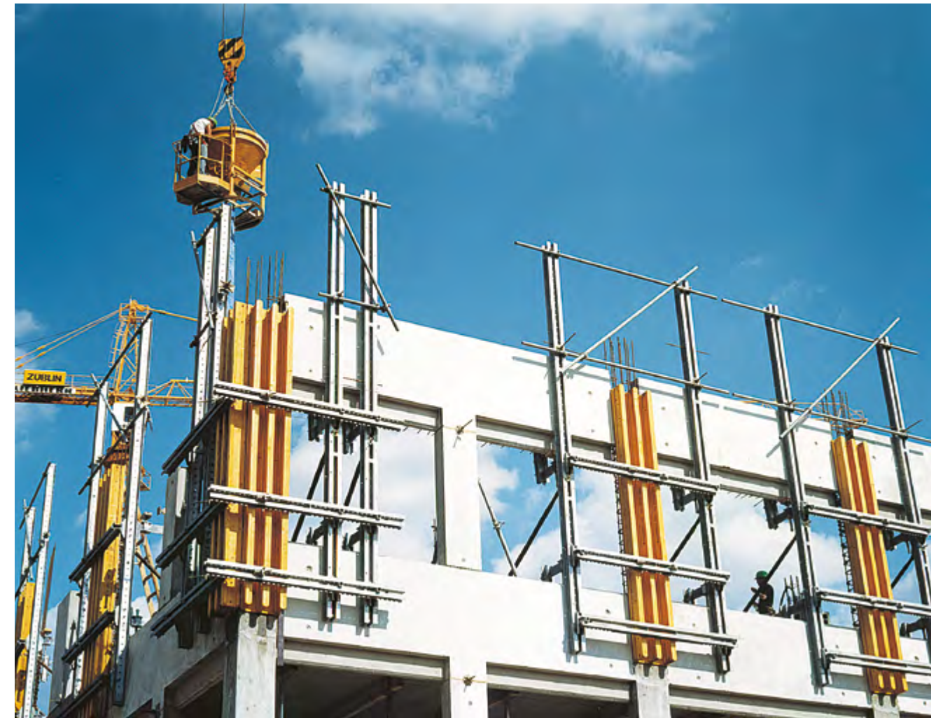
► The facade formwork enables mixed structures to be formed in economical procedures.
