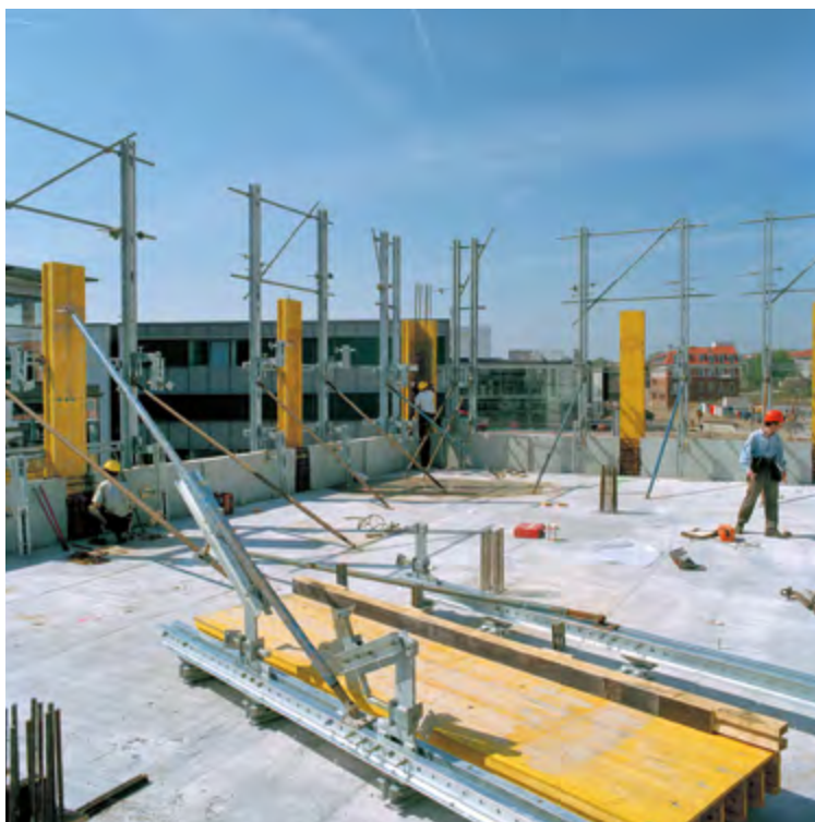
► Low quantities of equipment kept on site thanks to leading construction cycles
