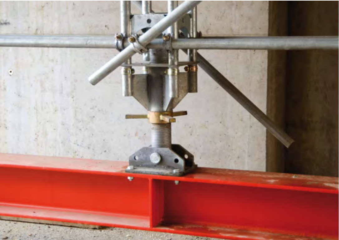
► Load-bearing frame props used as shoring solution for an unobstructed site underpass
