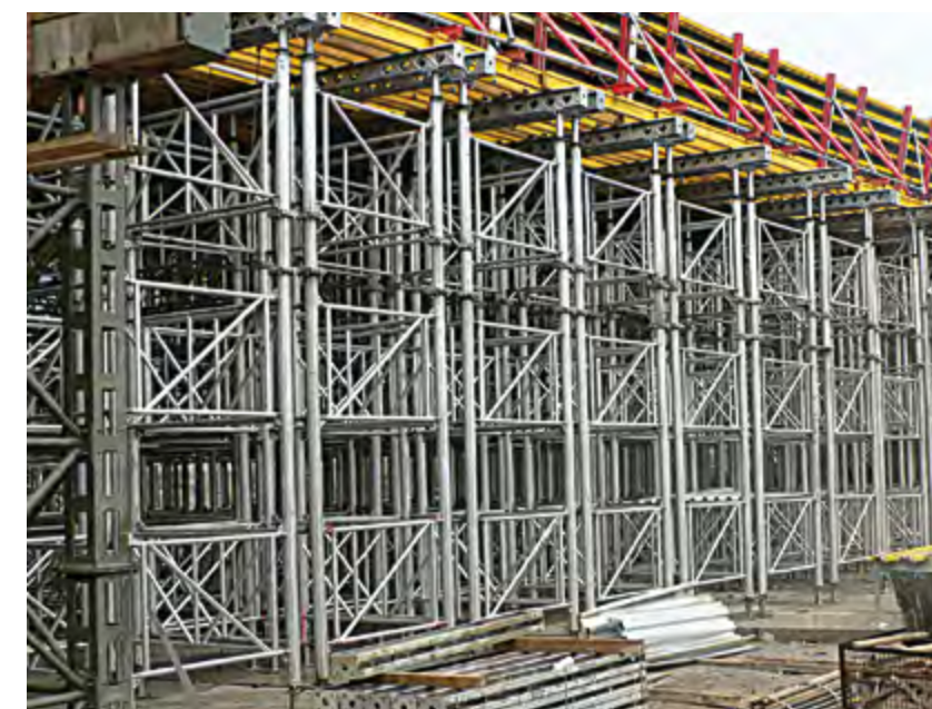
► Bridge deck and parapet shoring
