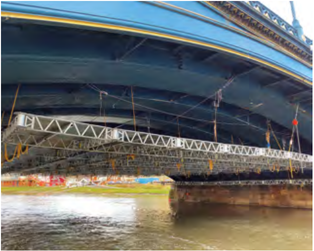
► Trent River Bridge (UK): QuikDeck provides large safety margins thanks to high load capacity of the suspension chains
