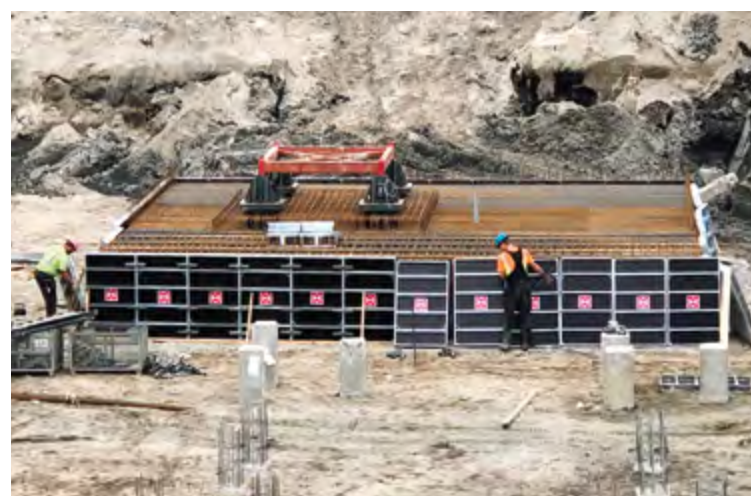
► Craneless forming possible due to low weight of basic RASTO panels
